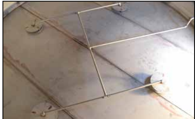
Fig 15 - Air injection diffusers
