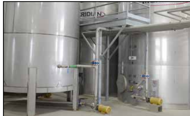
Fig 21 - Permanent fill and discharge system
