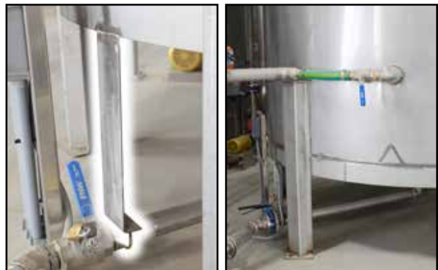
Fig 8 - Bracket to support piping from bottom coupler
